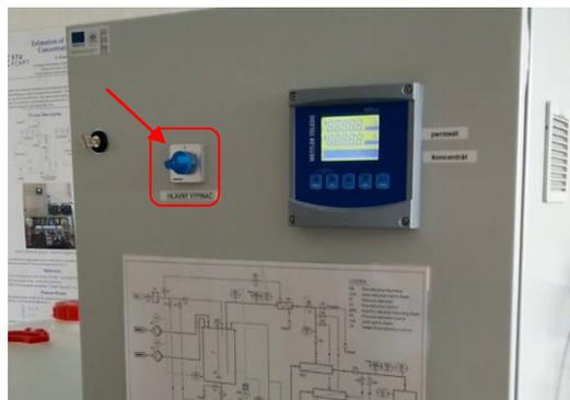
Picture 21 Flipping the switch (From 0 to I)
