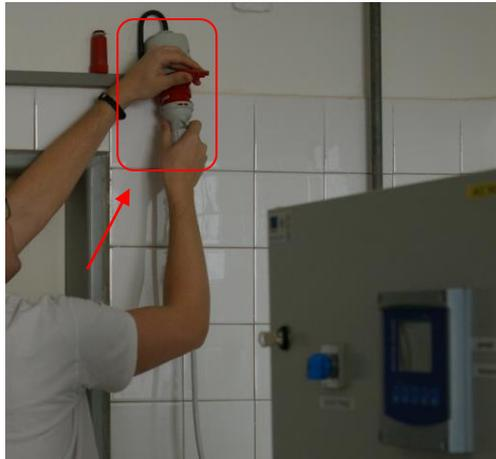
Picture 19 Plugging in the three-phase plug
