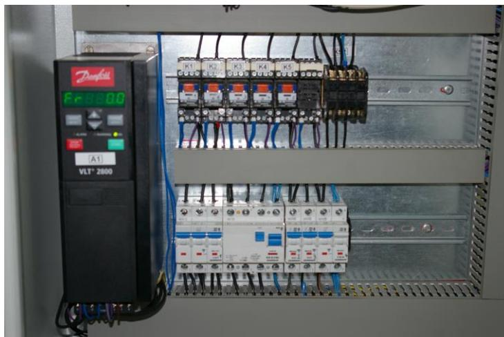
Picture 15 Danfoss VLT2800 frequency converter
